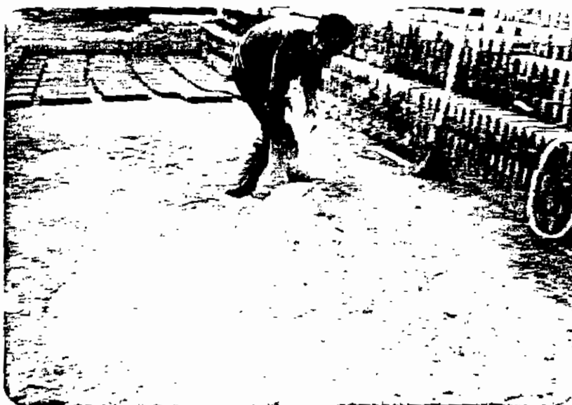
Fig. (8) Mixing Manually in Making Bricks in a Building Site.
