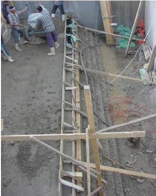
Fig. 19: Layering dam into 20 cm layers-thickness
