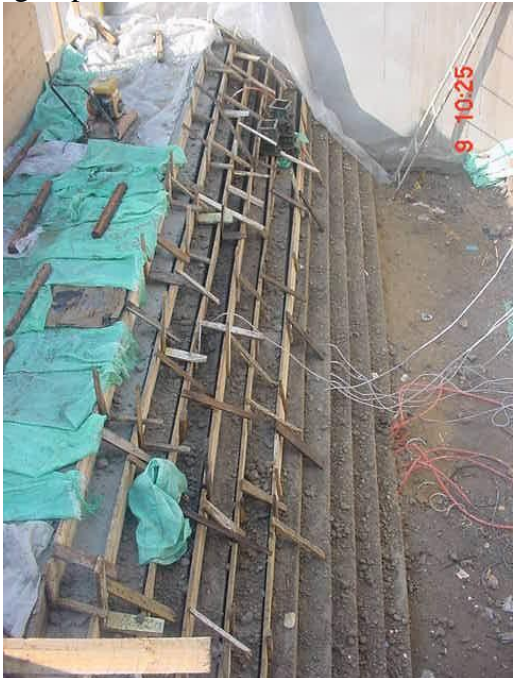
Fig. 23: Plastic covering for casted layers
