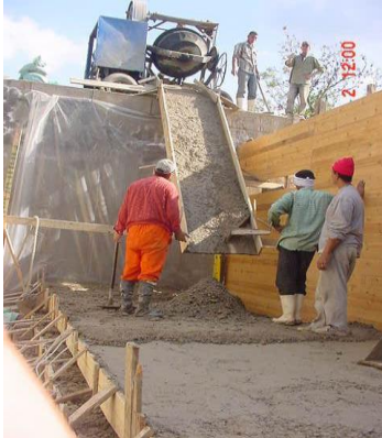
Fig. 17: Placement of concrete by gutter
