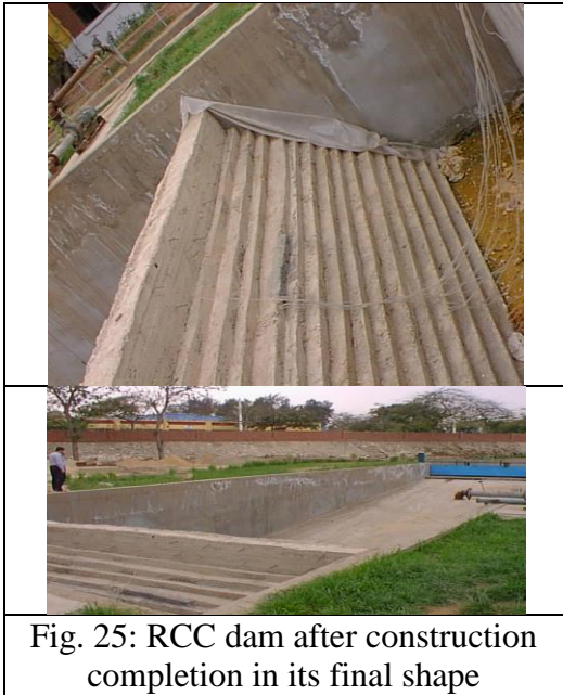
Fig. 23: Plastic covering for casted layers
