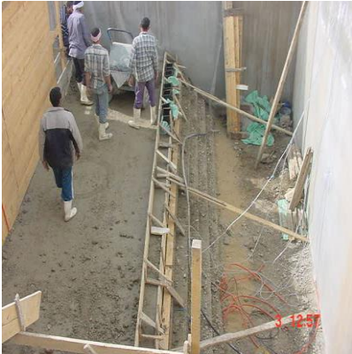
Fig. 20: Concrete placement into one of dam-layers
