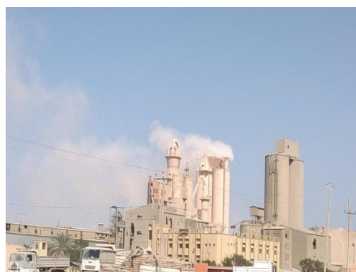
Figure (1) El-Mergheb Cement Factory
