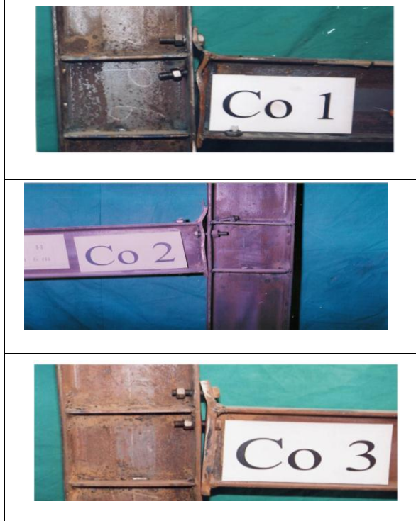
Fig. (25): Modes of Failure for the tested connections (Co.1, Co.2 & Co.3) in the group I
