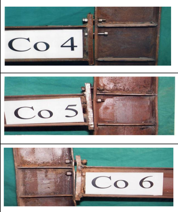
Fig. (26): Modes of Failure for the tested connections (Co.4, Co.5 & Co.6) in the group II
