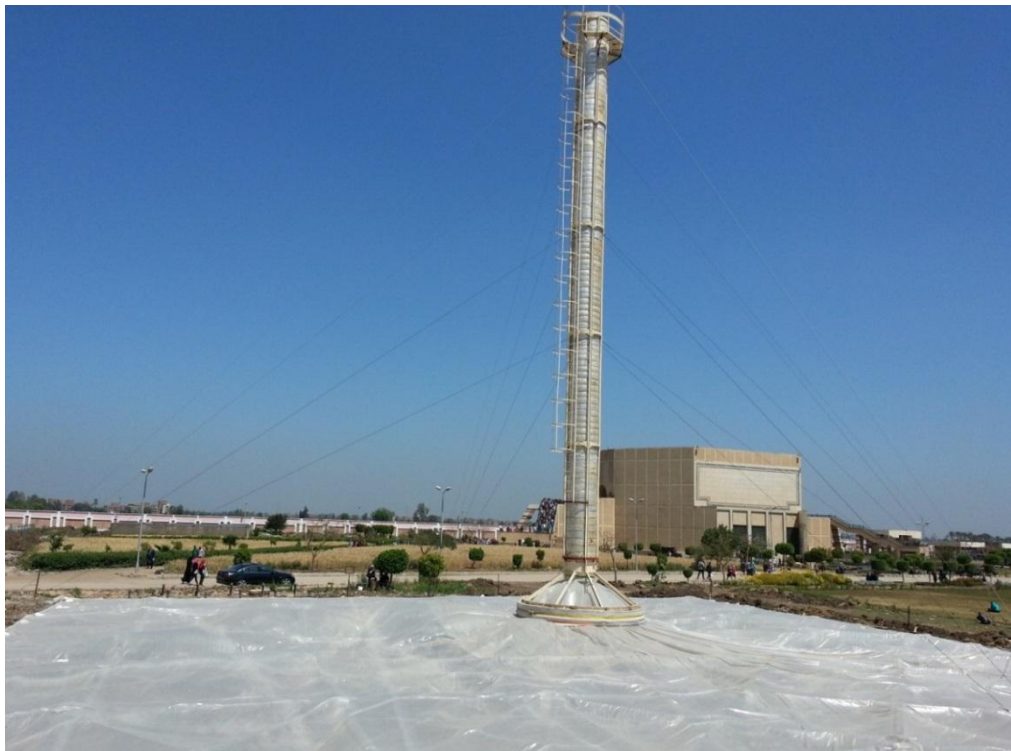
Figure 1 Photo of the experimental solar chimney pilot plant
