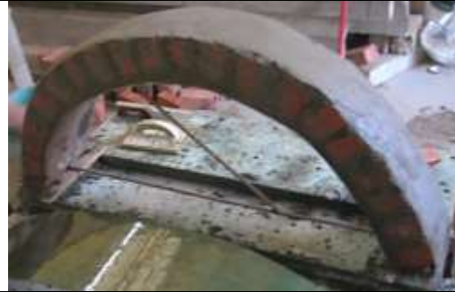
Figure 3: Construction of Semi-Circle Arch (S-Arch)
