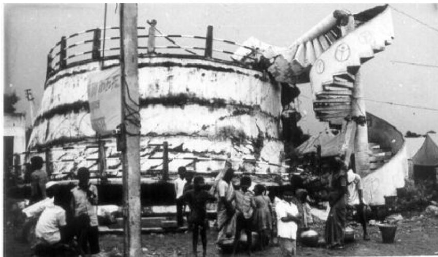
Fig.2 Collapsed elevated water tank in Killari 1993 earthquake
