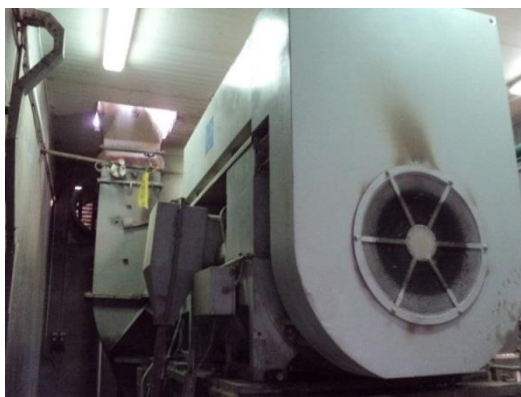
Fig. 2 Photographic image for atomization air blower
