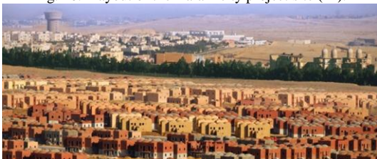
Fig. 11. Photo of Haram city project (11).
