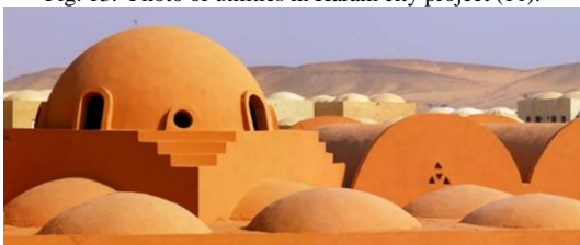
Fig. 14. Photo showing architectural style and building materials in Haram city project (11).
