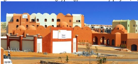
Fig. 13. Photo of utilities in Haram city project (11).
