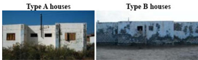
Fig.7. Photos of building typology of the Graduate Villages project site (10).
