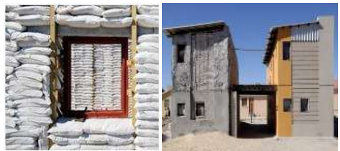
Fig. 12. Construction material of the Exterior wall
