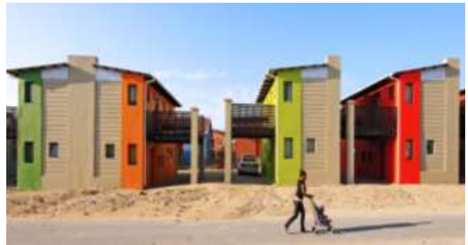
Fig. 11. Side view of sand bag housing project
