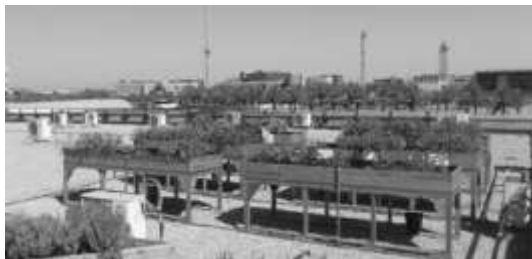
Fig. 3. Faculty housing's green roof. [16]
