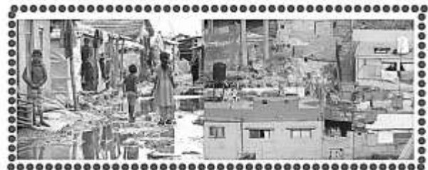
Figure 23: Deterioration of residential buildings and lack of
