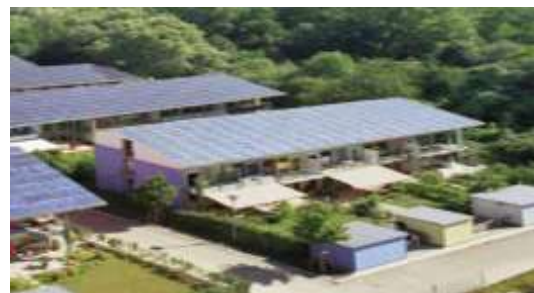
Fig. (12) Solar collectors on rooftops Source: ( https://www.mersinsolarwind.com/solar-paketler ) ( https://www.hethongnangluong.com/ )
