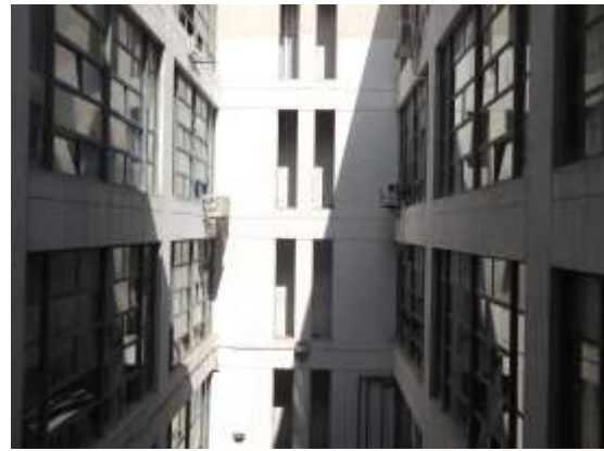
Fig. 19. Courtyard for secondary building. Source: Taken by the researcher on 15 Feb.
