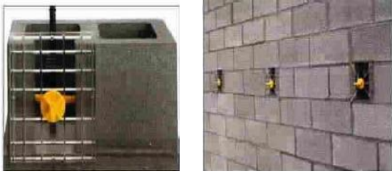
Fig. 6. the Transparent masonry grout clean
