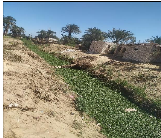
Photo (2): Unlined canal section
