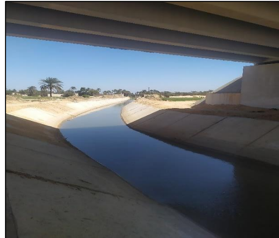
Photo (1): Lining works in the canal
