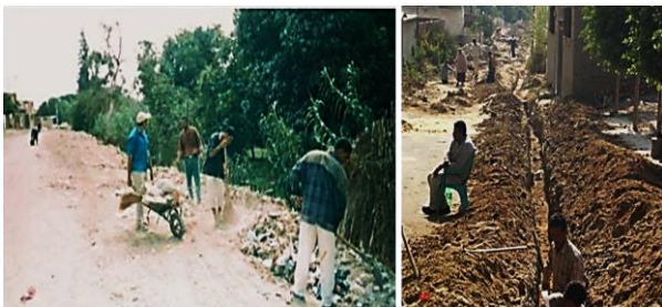
Figure.14: Physical upgrading of EL Bahtini (UNDP, 2011).
