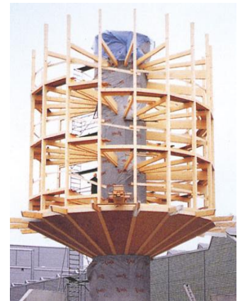
Fig (3):The wooden structure house at the time of execution
