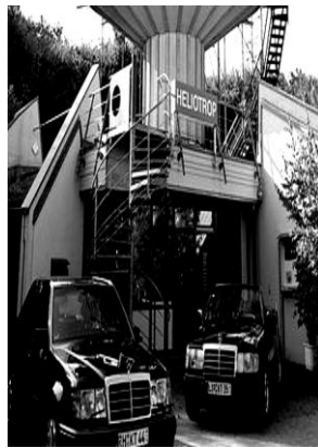
Figure (7): The main entrance of the dwelling in the ground floor
