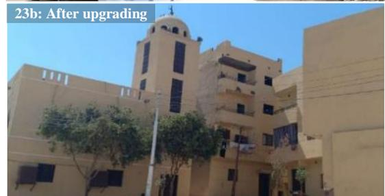
Fig. 23a and 23b. Building new parapets and walls to complete the missing parts (Photo credit: Authors)
