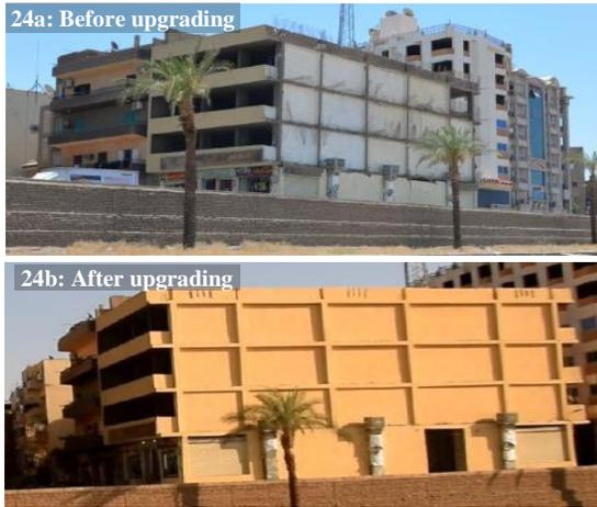
Fig. 24a and 24b. Finishing of the remaining parts of partially demolished buildings (Authors)
