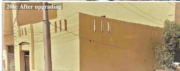
Fig. 20a and 20b. Unfinished walls were plastered and painted, and missing parapets were built (Photo credit: Authors)
