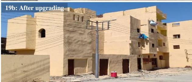
Fig. 19a and 19b. Irregular walls of unfinished façades were straightened in finishing phase (Photo credit: Authors)
