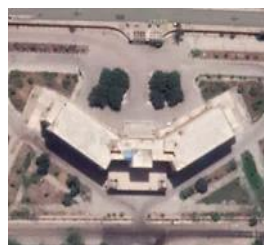
Fig (25) Top view of the building
