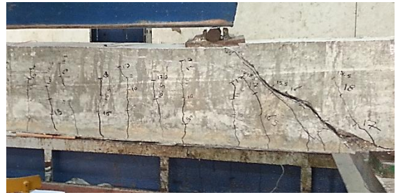
Fig. 7 Crack pattern of Beam BS01
