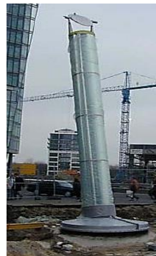
One of the lightpipes at Potsdamer Platz during installation
