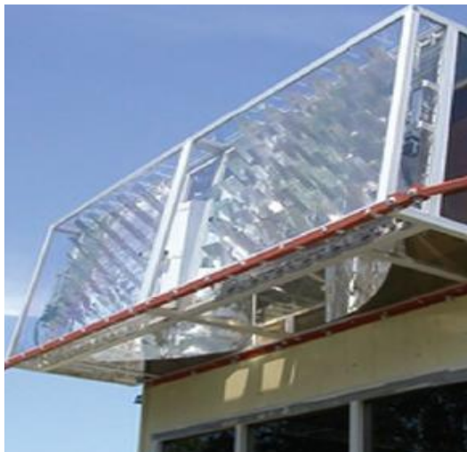
Solar Conopy Illumination System ( SCIS)
