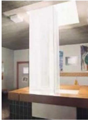
Light pipe, Heliobus system in Switzerland
