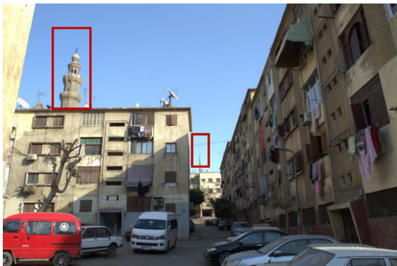
Fig. 8. The current situation of housing blocks that do not overview the surrounding ancient monuments in location (source: the authors).
