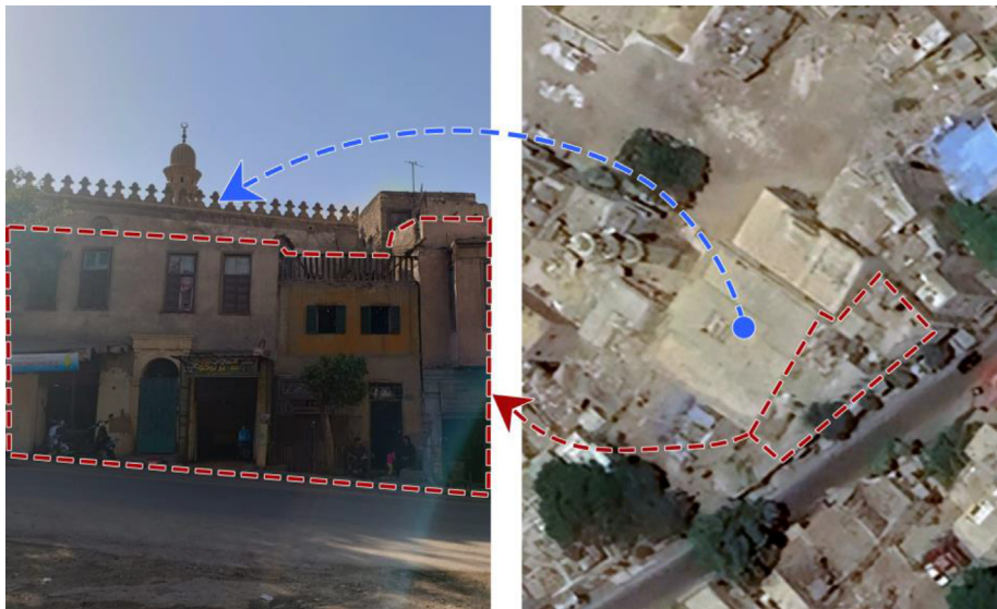
Fig. 11. Encroachments on the building's piece of land (source: the authors).
