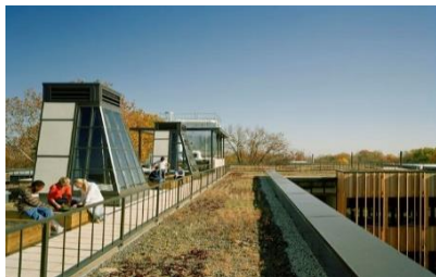
Figure 4: The solar chimney in roof. (AIA, 2007)
