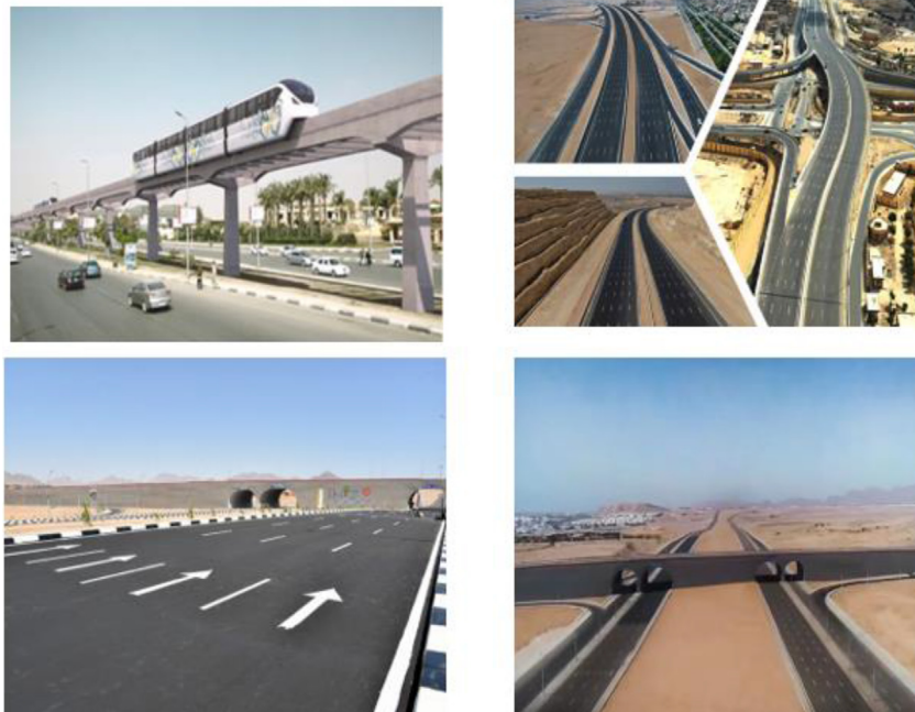
Fig. 12. Photos of several road development projects in Egypt ( https://images.app.goo.gl/qr9Q3L3CmAMtzUcK9 ).
