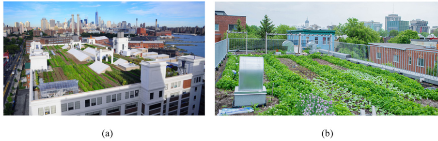
Fig. 2. Rooftop soil farm examples. (a) Brooklyn Grange rooftop farming and intensive green roofing in the United States (b) The Roulant's roof garden, Montreal, Canada. Source (Hsieh et al., 2018).
