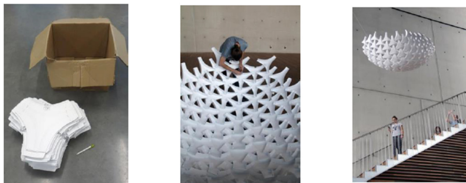
Fig. 11. The assembly process of Undulatus pavilion hanging at the IASS2015 expo (Brancart et al., 2015).
