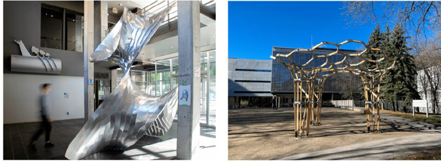
Fig. 1. Topologies of lightweight constructions (Left) continuous shell (Right) discretized shell (Nejur, 2023).
